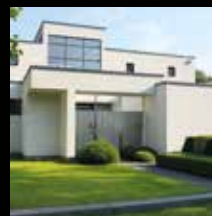
Find insulation problems
